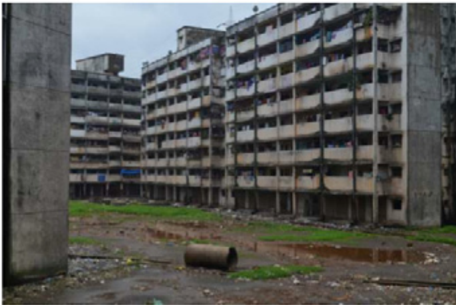
Figure 5: G+7 replacement housing for slums in M-East Ward, Mumbai with mixed use provisions in the ground floor which remain unallotted. Source: ACE 2014
