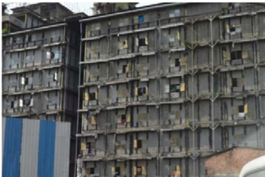
Figure 6: High-rise EWS housing in the peripheries of a private development in Mumbai. Source: ACE 2014
